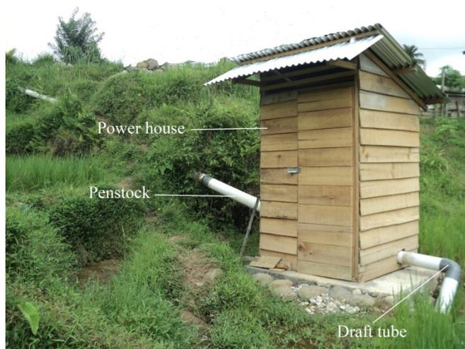
Fig. 6. Photo of power house for securing test equipment.
